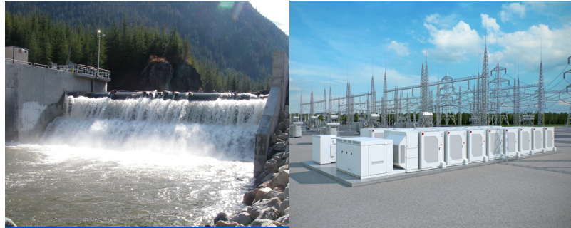
100MW Run-of-River Hydro Plant + 50MW Battery Participate with 70MW in Capacity/Peaking Market and with 100MW in Energy Market
