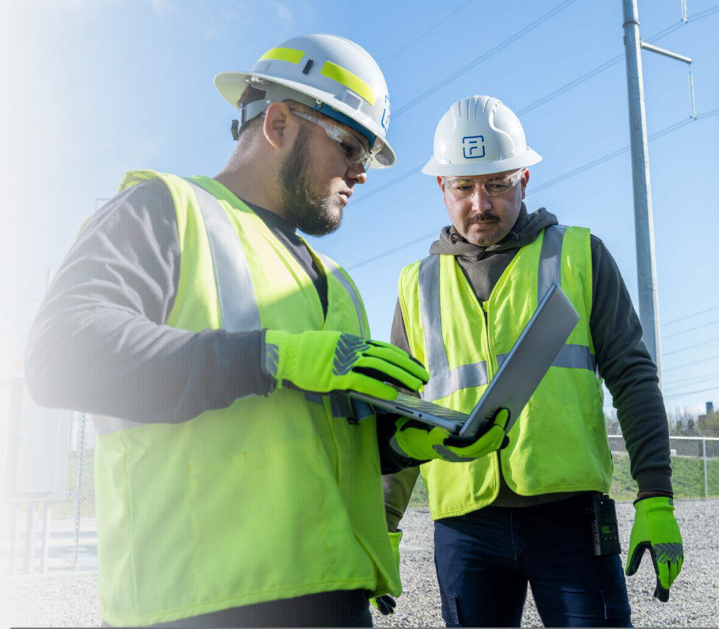
Caption: Project team members at the Pike County Battery Energy Storage System in Indiana, with more than 1,300 Fluence Gridstack systems delivered and installed from our Utah production facility.
