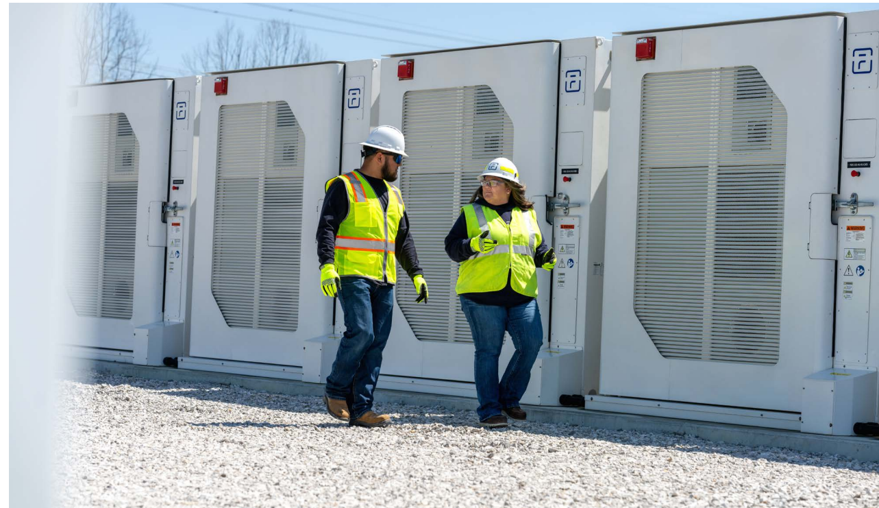
Caption: Project team members at the Pike County Battery Energy Storage System in Indiana.
